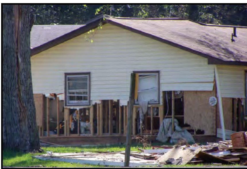
A structure damaged by a Hurricane.
