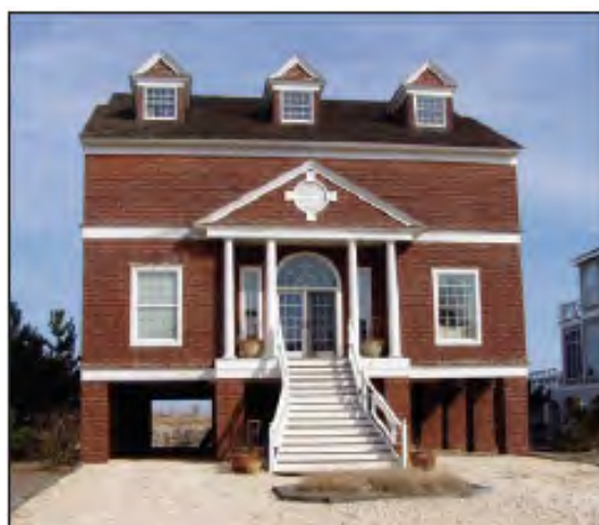
Coastal home elevated to avoid future flooding.
