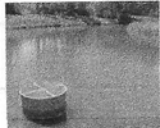
Retention Pond in North Carolina
