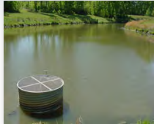
Retention Pond in North Carolina
