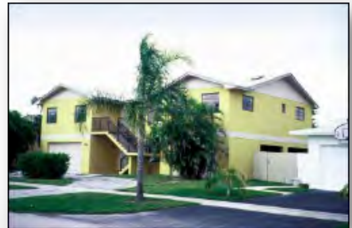
Top Picture: A house in Miami in the process of being elevated.
