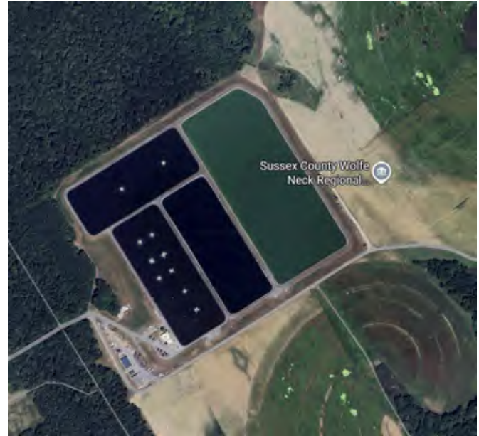
Wolfe Neck Regional Wastewater Facility
