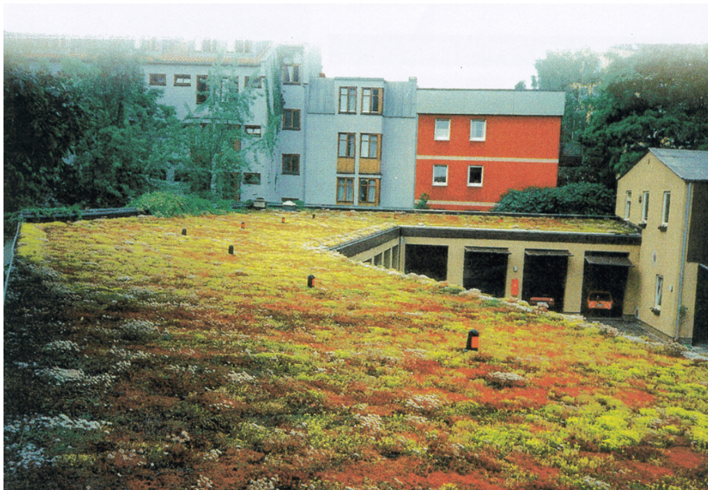
An example of a green roof, with vegetation over vehicle garages in an apartment complex.
