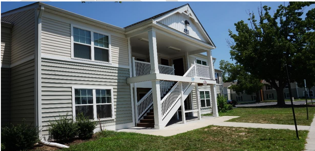
Figure 18. Meadowbridge Apartments, Seaford, Delaware Received Low-Income Housing Tax Credits to finance a complete renovation in 2017. The property has 104 units all affordable to households earning up to 60% of the area median income.
