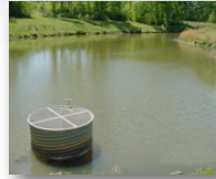
Retention Pond in North Carolina
