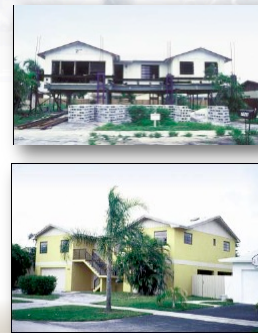
Top Picture: A house in Miami in the process of being elevated. Bottom Picture: That same house once completed. Taken from FEMA, Above the Flood, 2000
