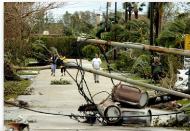
Fallen utility lines after Wilma. From www.galtmile.com
