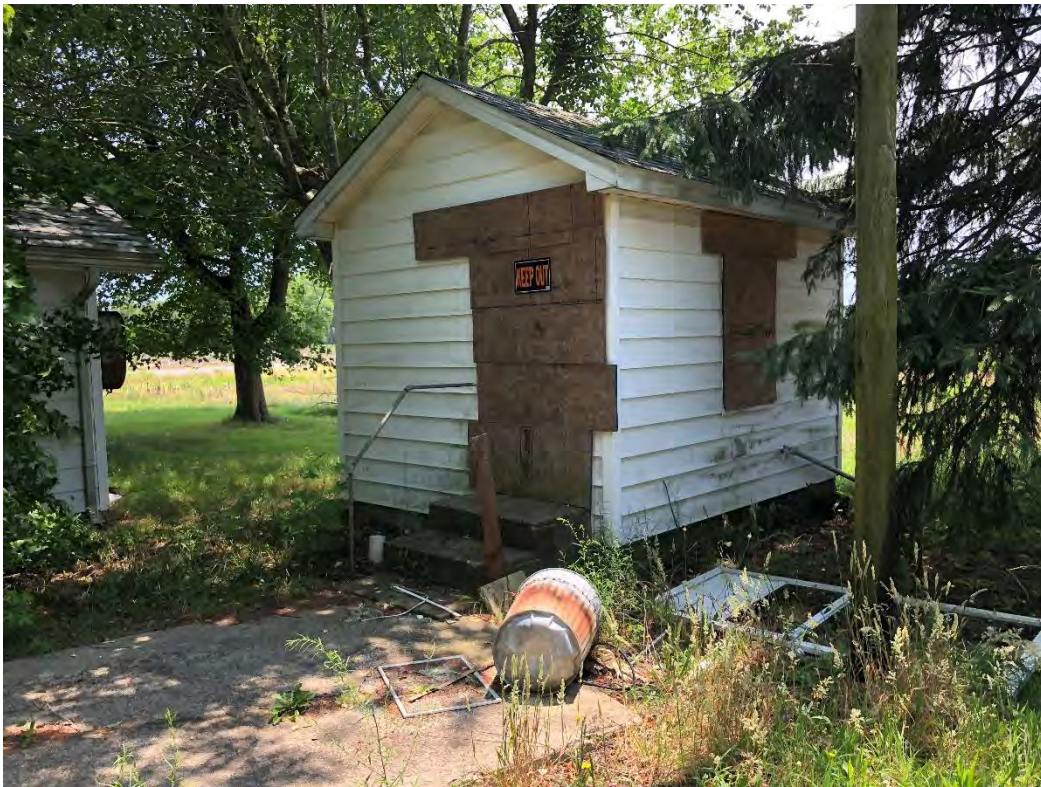
Photo 4: Outbuilding at Residence
