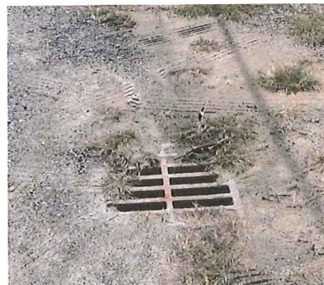
Catch Basin at River View Avenue
