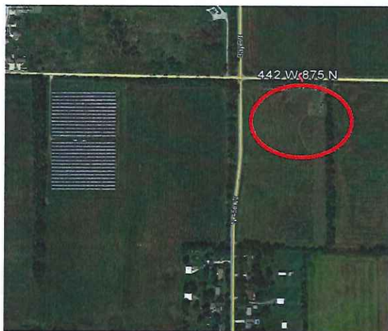
Portage Solar Farm, IN October 2015
