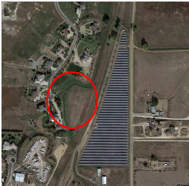
Brighton PV Solar, Adams County, CO June 2016
