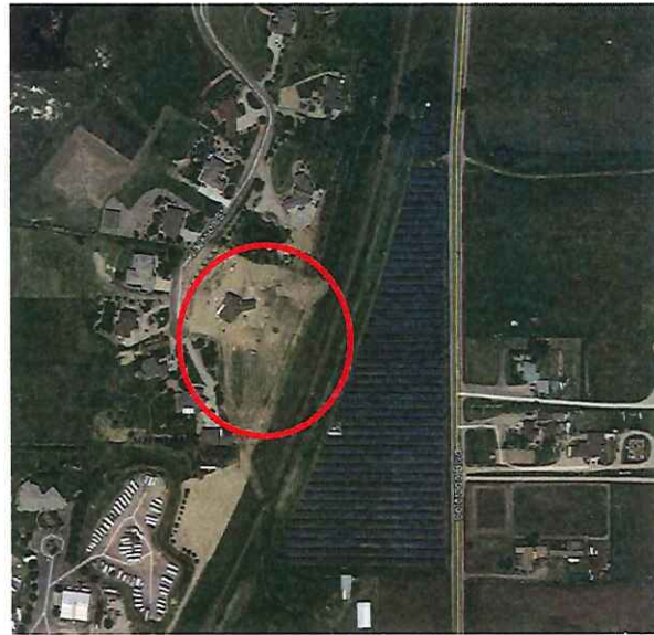
Brighton PV Solar, Adams County, CO June 2017
