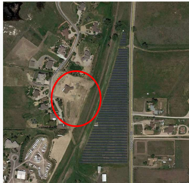
Brighton PV Solar, Adams County, CO June 2017
