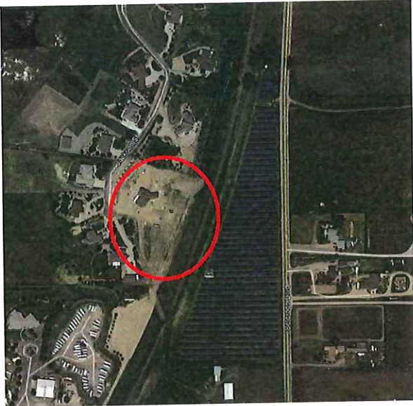
Brighton PV Solar, Adams County, CO June 2017
