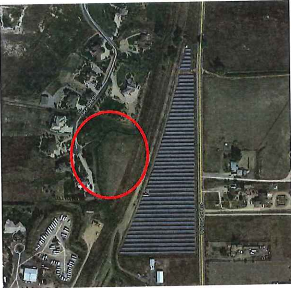
Brighton PV Solar, Adams County, CO June 2016
