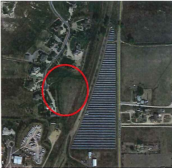
Brighton PV Solar, Adams County, CO June 2016
