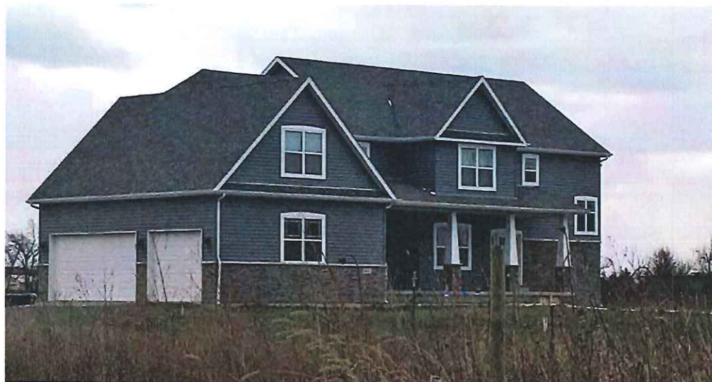
4,255 square foot estate home under construction, adjacent to Portage Solar Farm located in Indiana
