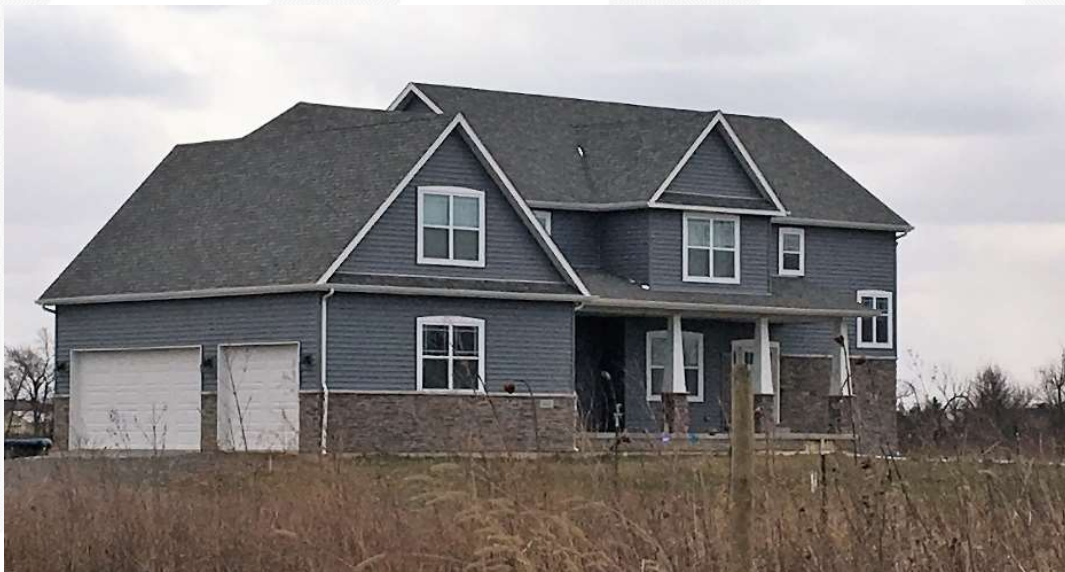
4,255 square foot estate home under construction, adjacent to Portage Solar Farm located in Indiana On-site pond and attached garage (cost estimated at $465,000) April 2018
