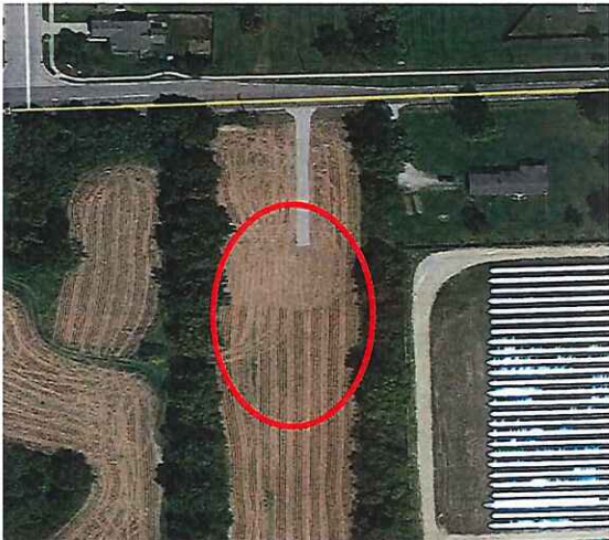
Dominion Indy III Solar Farm September 2014
