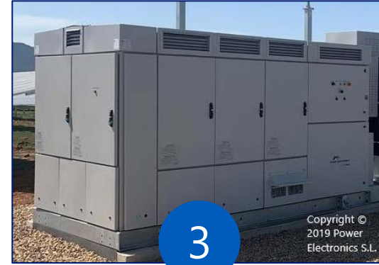
Inverter/Transformer Skid
