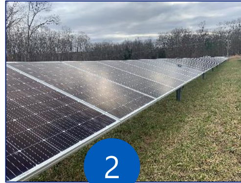
Panels installed on racking
