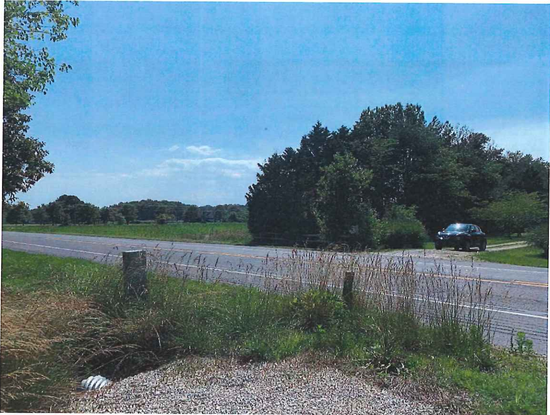
The Parler's entrance (where car is shown) is approximately 25'-0" from the proposed entrance of the commercial development facility (to the left of tree line) creating a hazardous access to the Parler's lane
