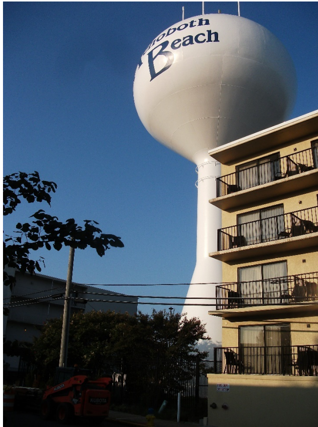
7. Site example showing the elevated storage tank proximity to The Breakers Hotel and 2 nd Street, in Rehoboth Beach.
