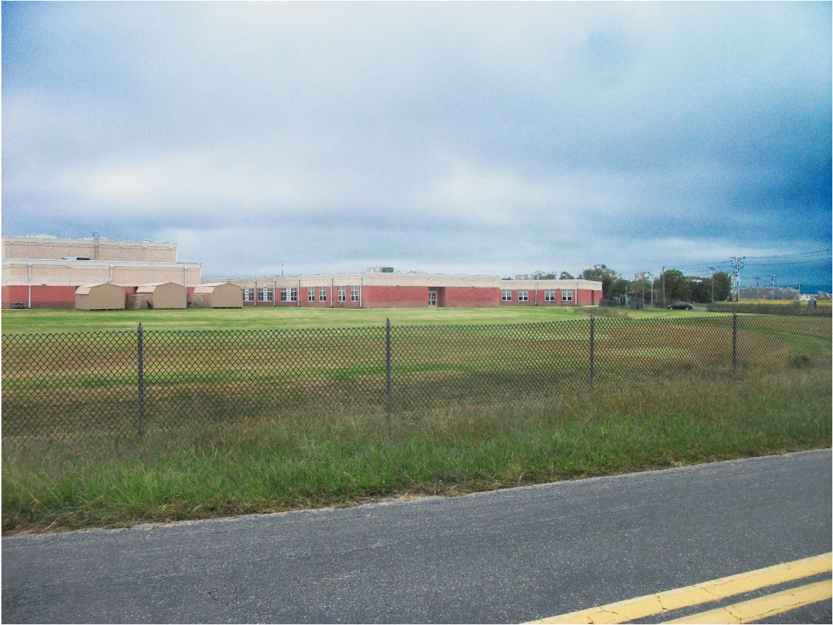
5. Looking northwest toward the proposed elevated storage tank location from Mulberry Knoll Road.
