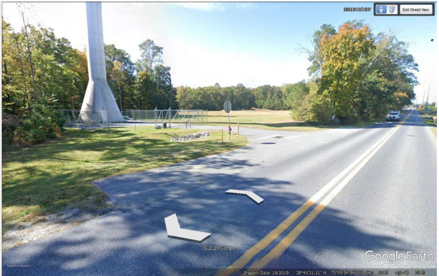
13. Example of existing Tidewater Utilities, Inc. elevated storage tank with approved DeIDOT entrance.
