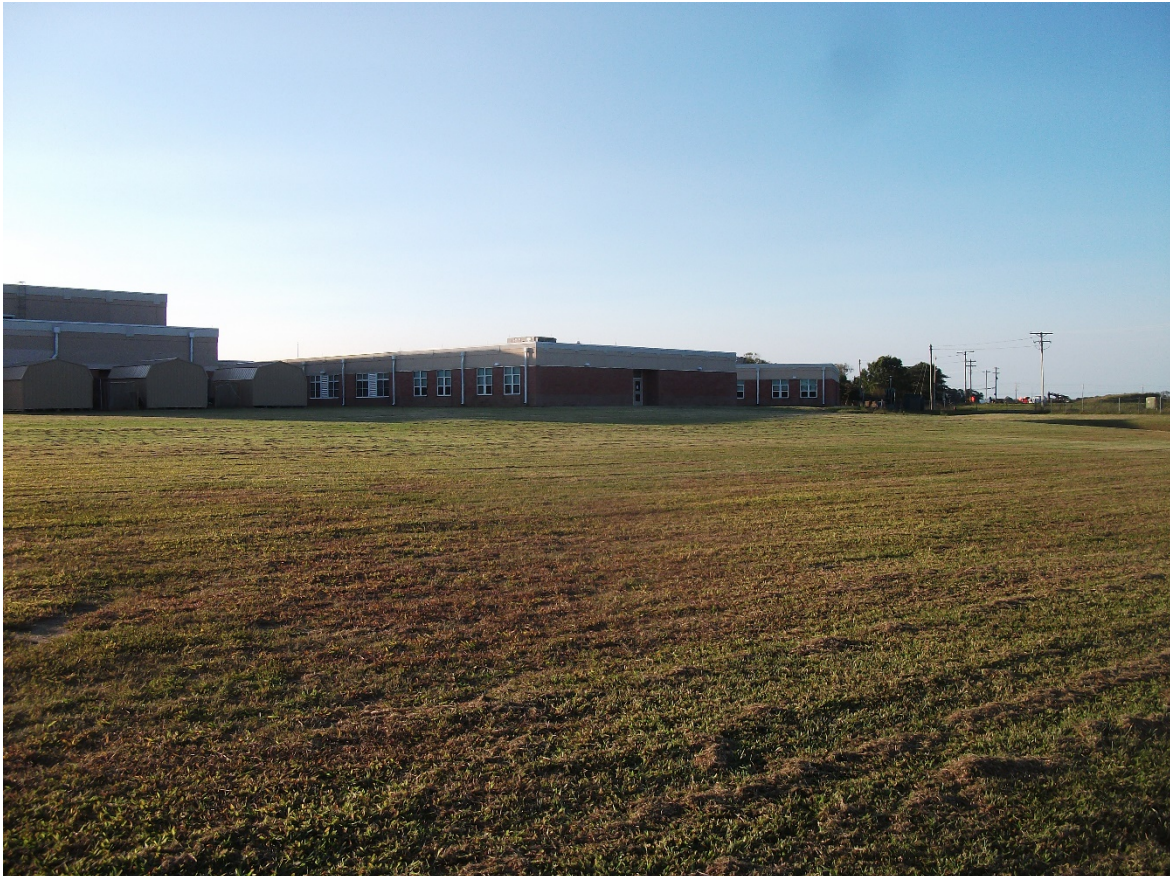
2. Looking northwest past the proposed elevated storage tank location, west of Mulberry Knoll Road.
