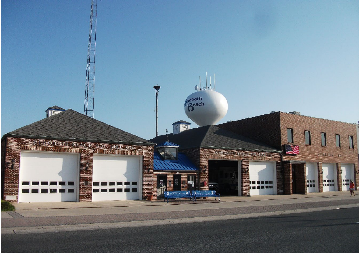
12. Site example looking north towards the water spheroid from Rehoboth Avenue, in Rehoboth Beach.
