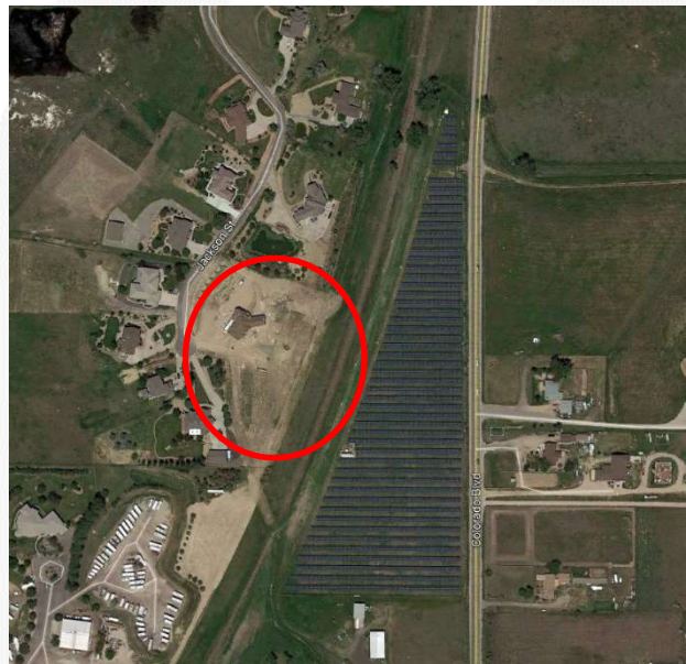
Brighton PV Solar, Adams County, CO June 2017
