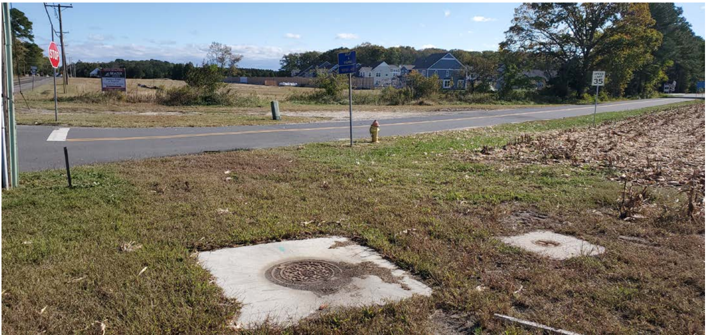
October 18, 2019 - Corner of Sand Cove Road and Route 54 Sussex County sanitary sewer manhole and cleanout have been installed Artesian Water Company Fire Hydrant has been installed
