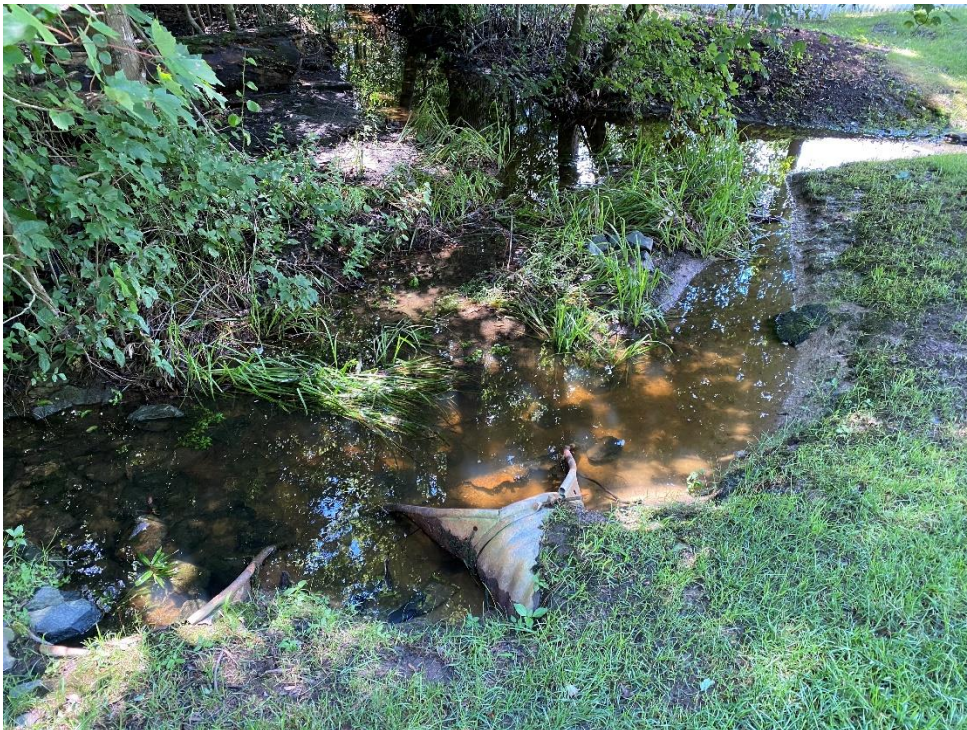
Photo 2: Sarah Run in Pipe Under Aintree Drive.
