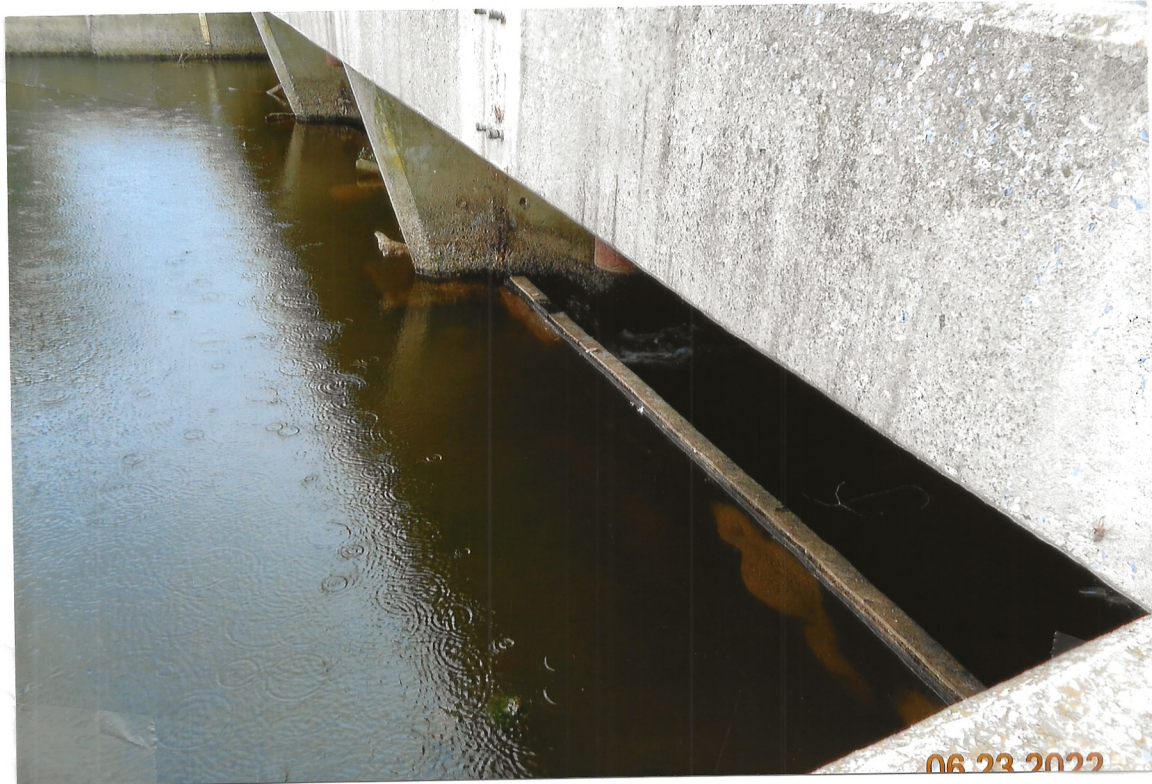
Figure 2. Photograph of the dam at the western end of Ingram Pond, Millsboro, Sussex County, Delaware. The dam obstructs the inflow or outflow of water into/out of the pond.
