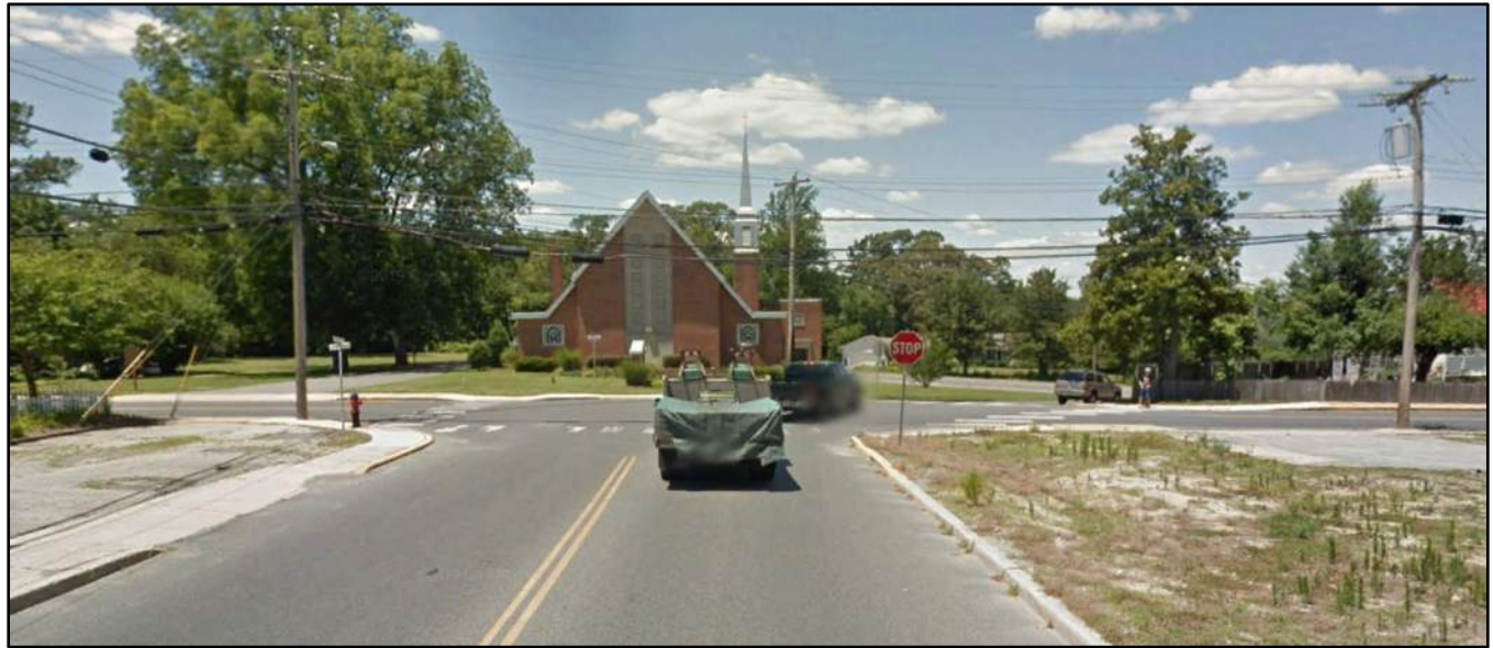
8_Delaware Route 5 and Mulberry Street (SR 197) / Atlantic Street (SR 88) Westbound Atlantic Street (SR 88) Approach
