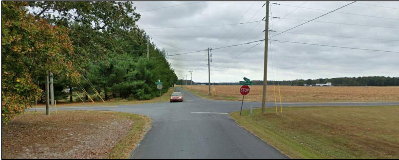
5_Pettyjohn Road (SR 255) and Prettyman Road (SR 254) Northbound Pettyjohn Road (SR 255) Approach
