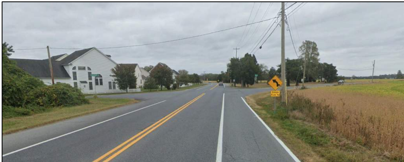
6_Delaware Route 5 and Shingle Point Road (SR 249) Southbound DE Route 5 Approach
