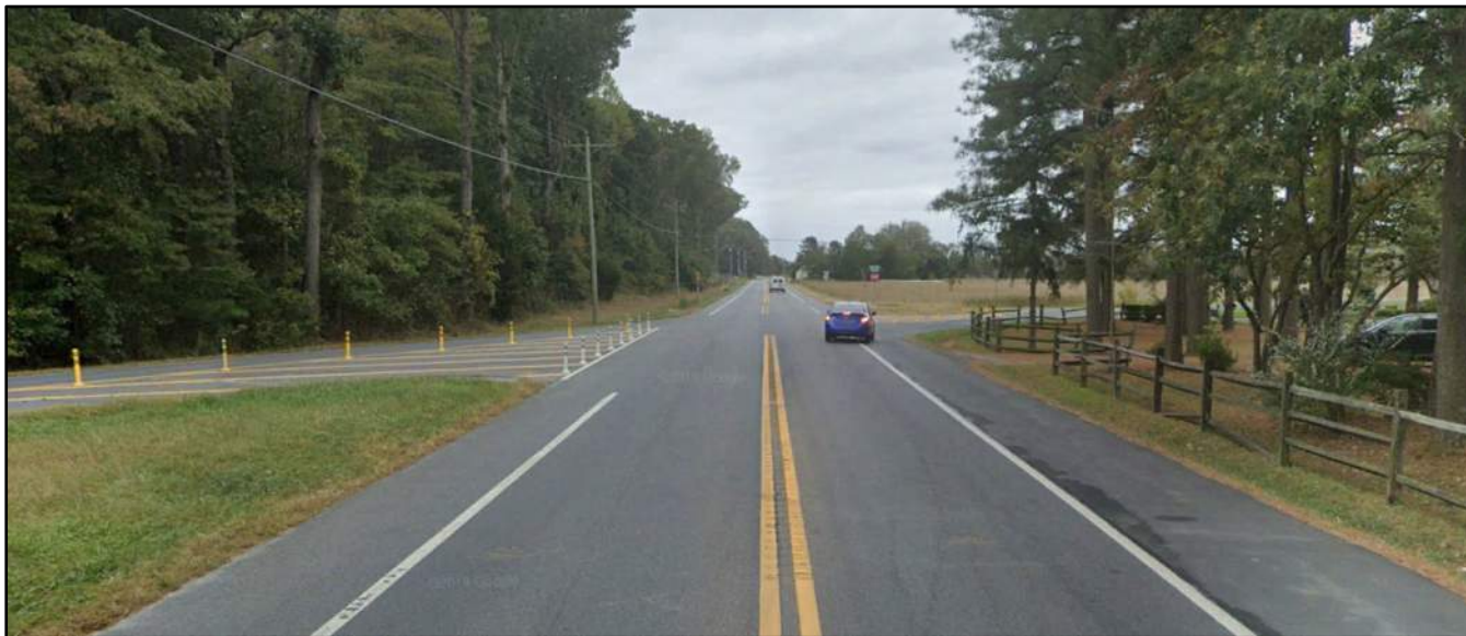
1_Delaware Route 30 and Shingle Point Road (SR 249) Southbound Delaware Route 30 Approach
