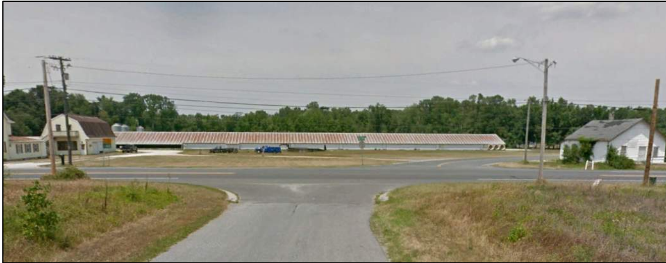
3_US Route 9 and Shingle Point Road (SR 249) Northbound French Road Approach
