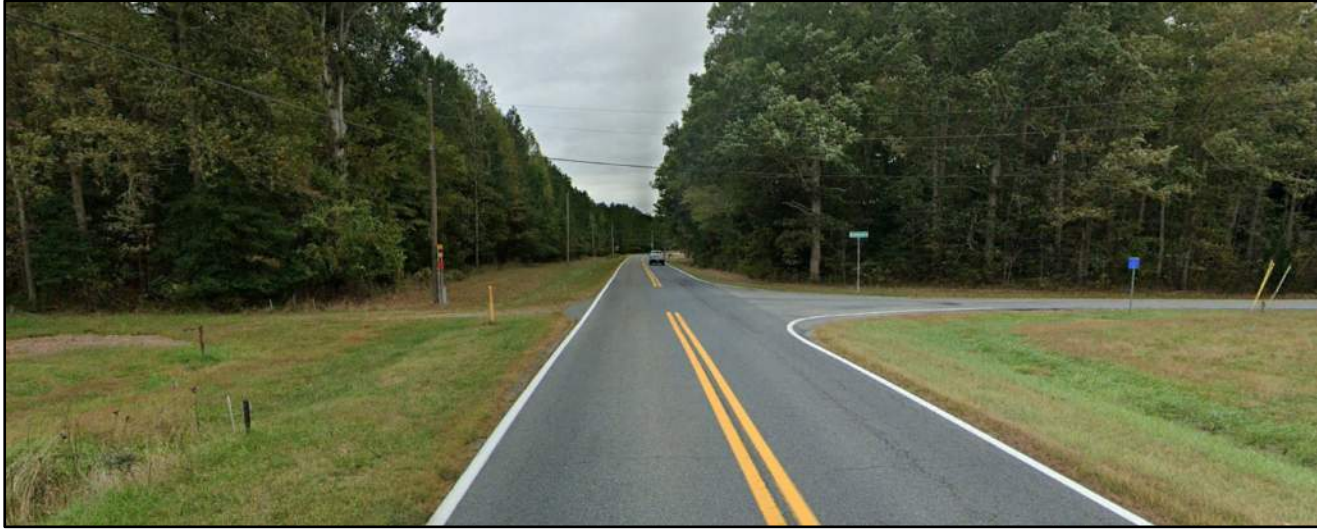
2_Shingle Point Road (SR 249) and Briarwood Road (SR 253) Southbound Shingle Point Road (SR 249) Approach
