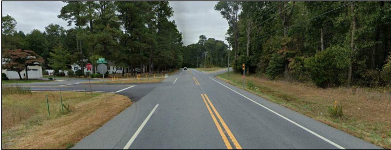
1_Delaware Route 30 and Shingle Point Road (SR 249) Northbound Delaware Route 30 Approach
