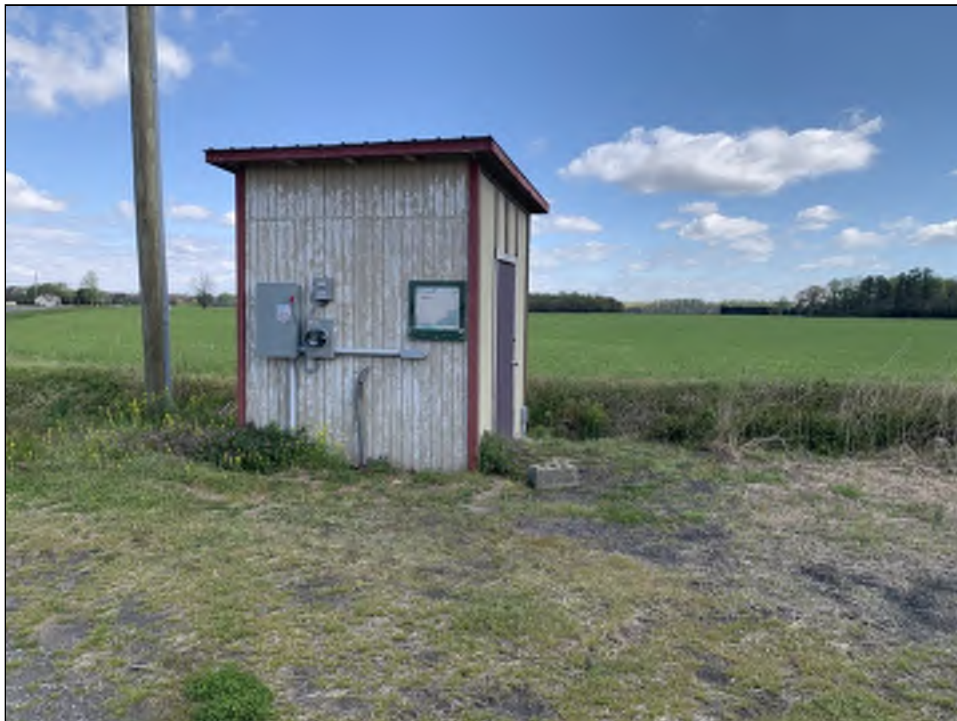
Photograph 14: View of Pumphouse
