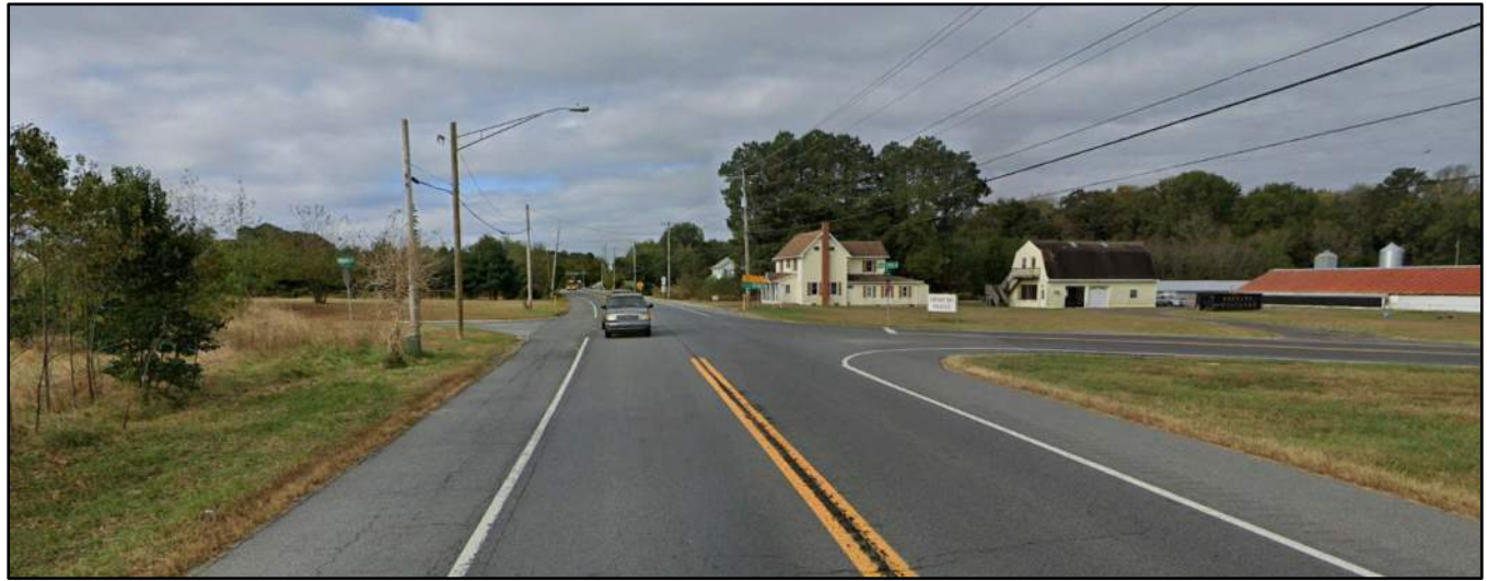
3_US Route 9 and Shingle Point Road (SR 249) Westbound US Route 9 Approach
