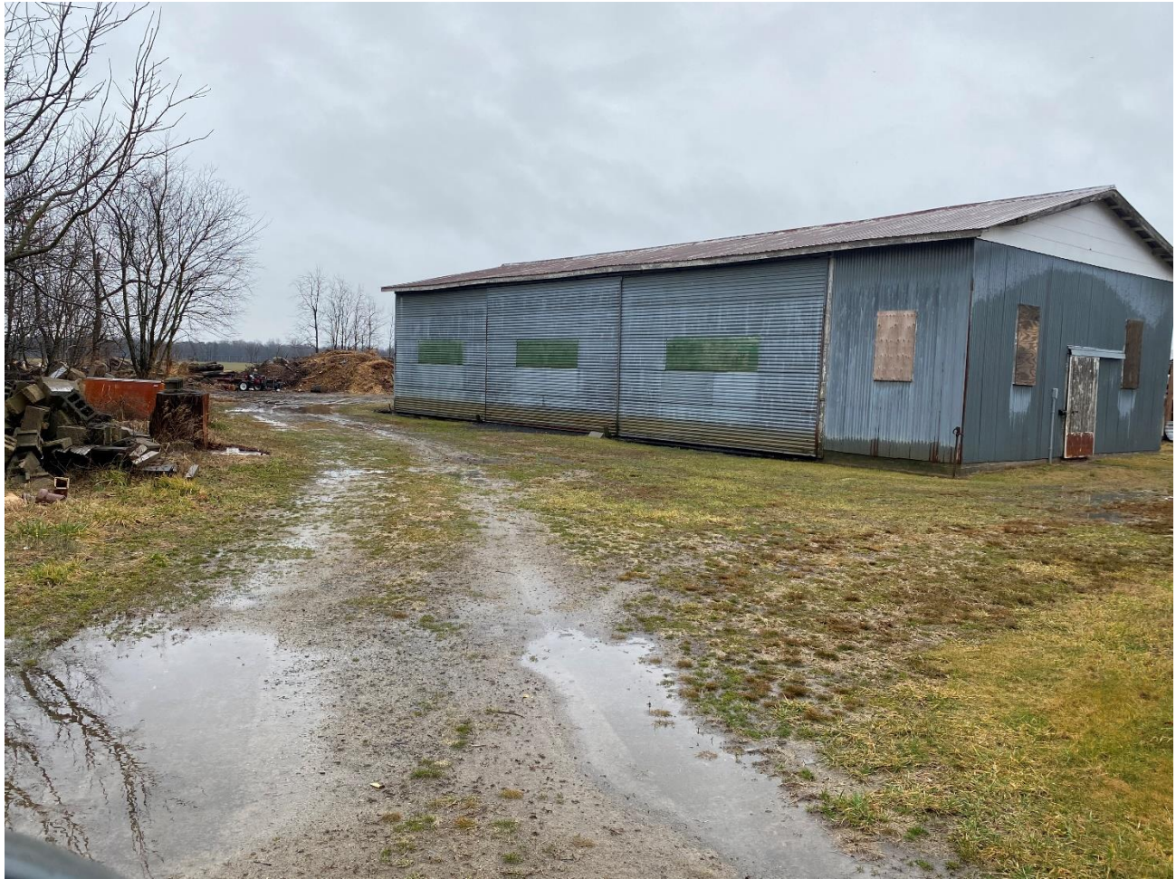
THE SECOND OF TWO BUILDINGS LOCATED ON THE NORTHEAST CORNER OF THE PROPERTY.
