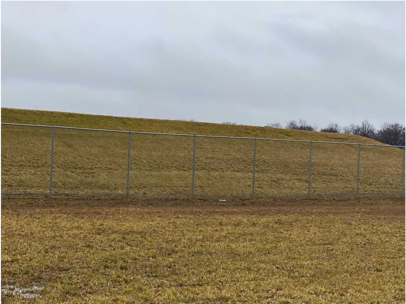
A PORTION OF THE EARTHEN BERM WHICH FORMS THE LAGOON WALL ALONG WITH THE SECURITY FENCE WHICH SURROUNDS IT.
