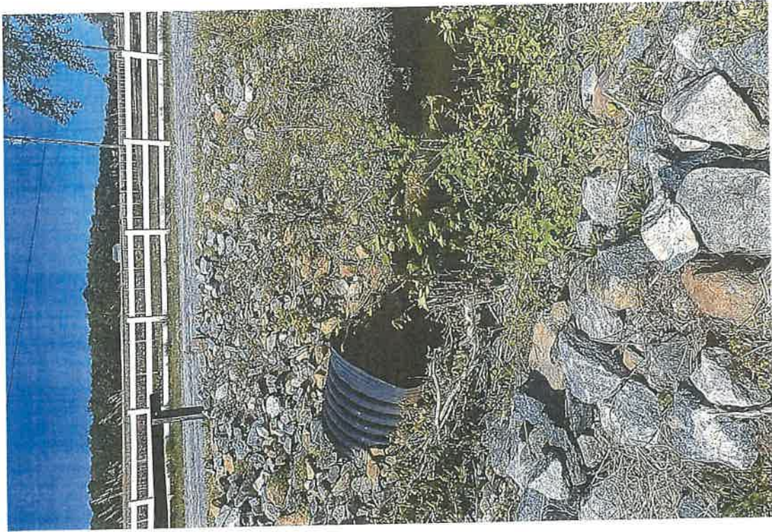
Photo 5 TAX Ditch Culvert under Horse Play way
