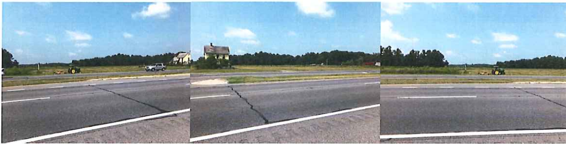
Site work being completed, July 2021.
