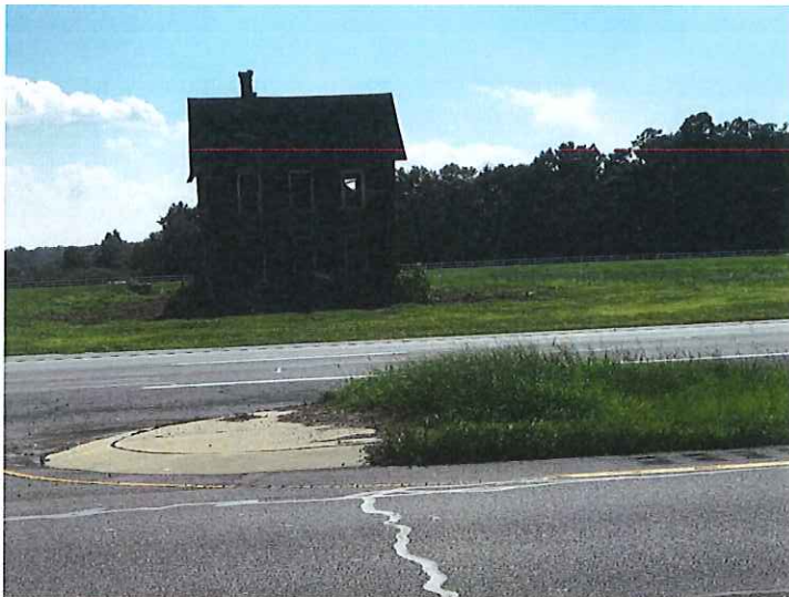
House following clearing and asbestos removal, August 2021.
