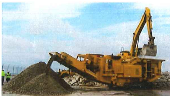
Crushing machine being loaded with construction debris by an excavator.
