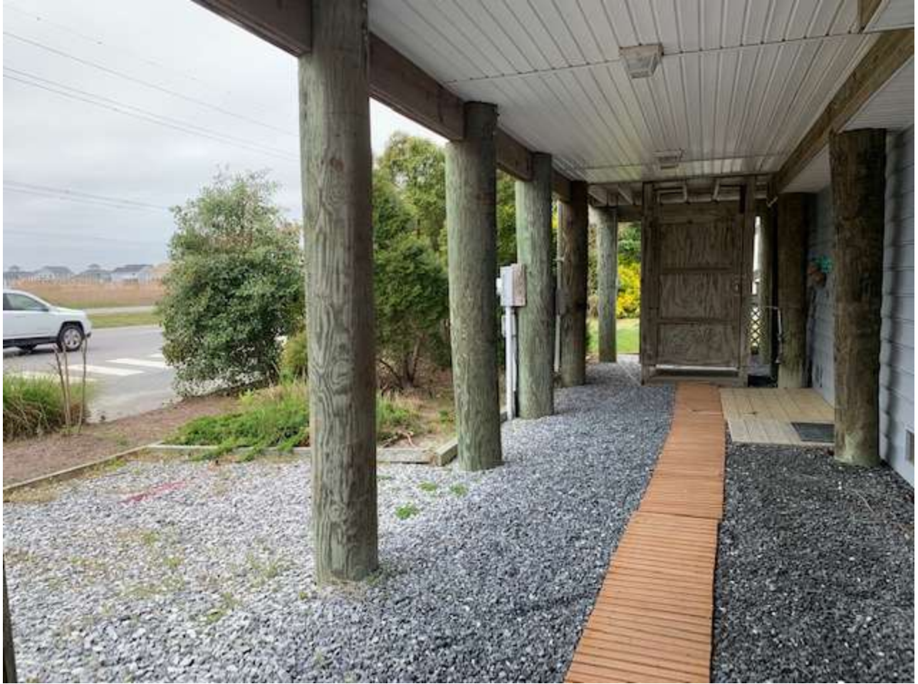
Side of house, side door and shower facing the highway
