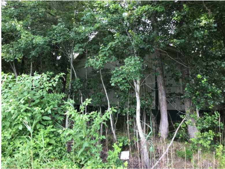
PHOTOGRAPH 5: Apparent wastewater treatment structure on the northcentral portion of the site.
