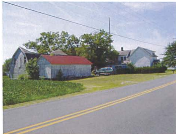
Existing dwelling located south of Railway Road.
