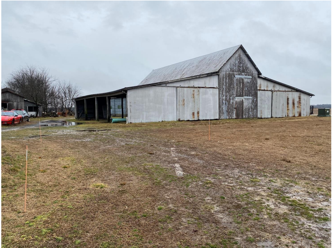
ONE OF THE TWO EXISTING BUILDINGS LOCATED ON THE NORTHEAST CORNER OF THE PROPERTY.
