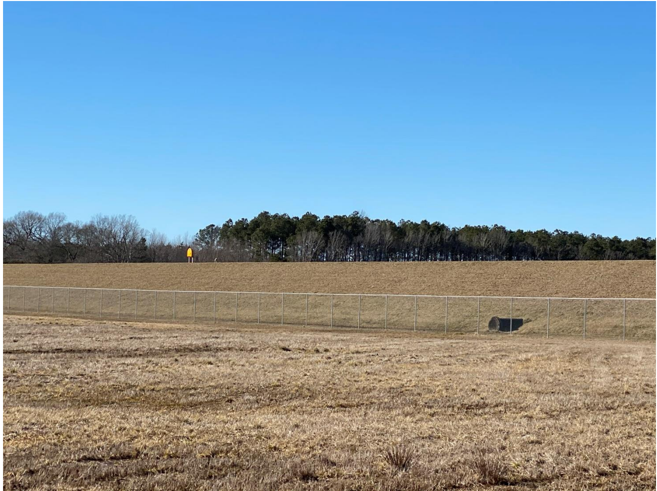
THE SOUTHWARD FACING LAGOON WALL AS SEEN FROM THE INTERNAL ROAD ON THE SRRF PROPERTY.
