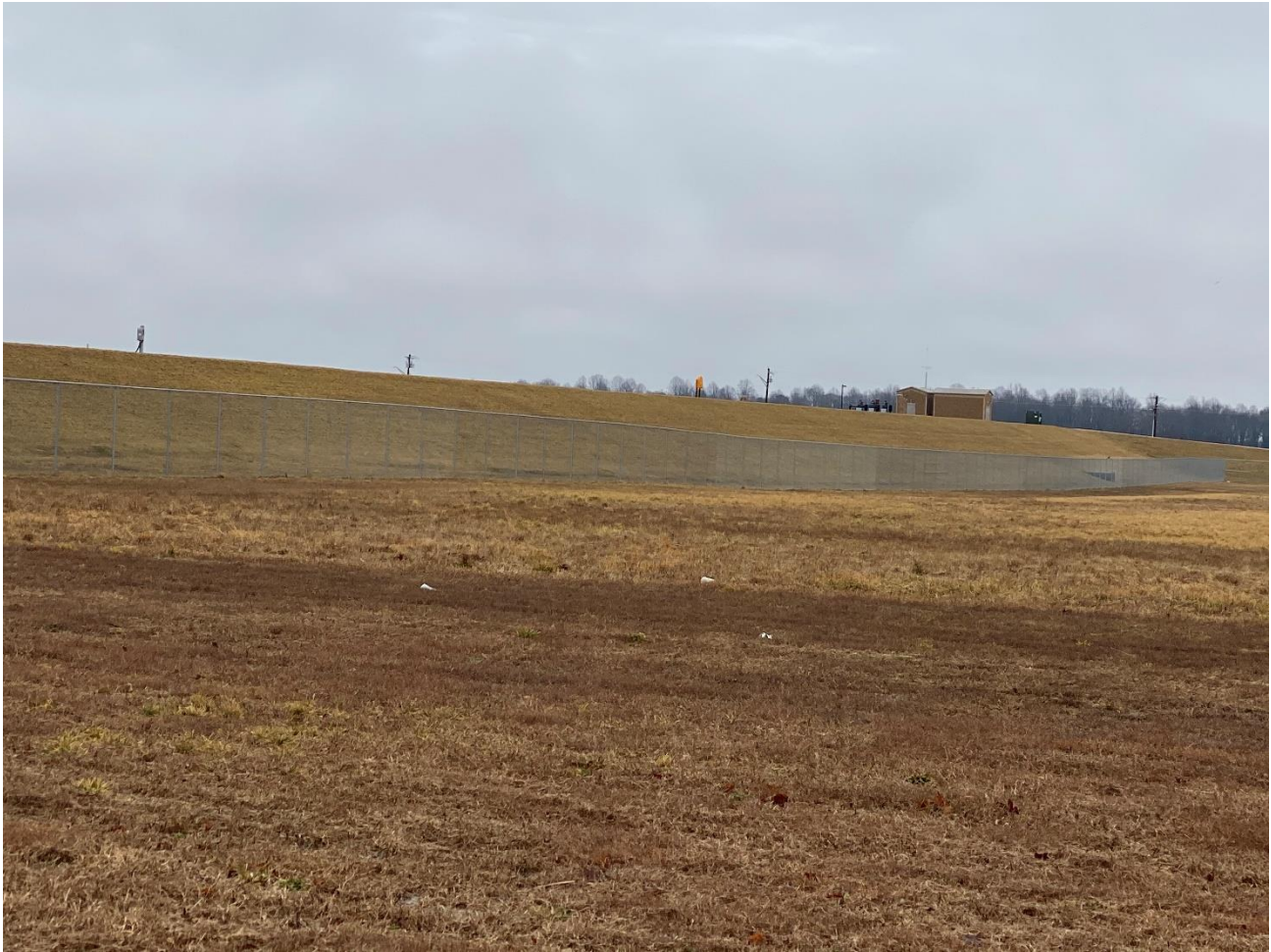
THE SOUTHWARD FACING LAGOON WALL AS SEEN FROM ROUTE 30.
