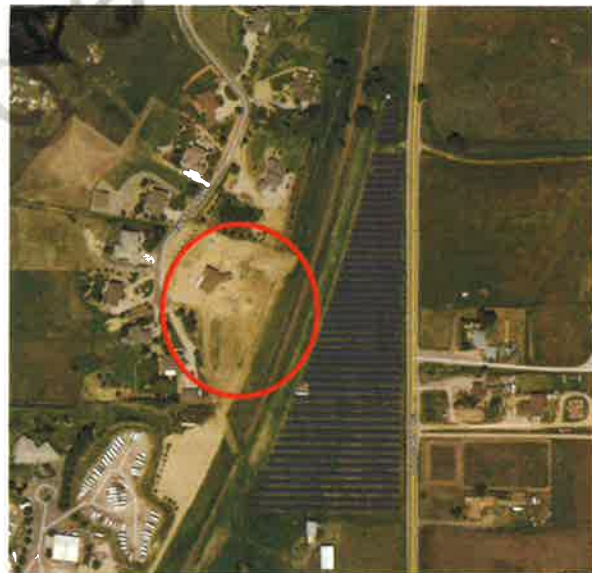
Brighton PV Solar, Adams County, CO June 2017
