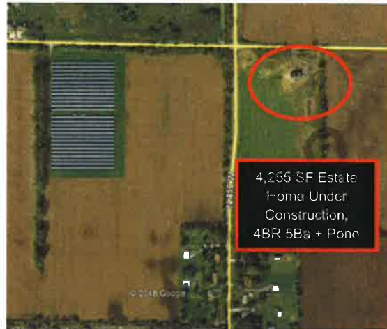
Portage Solar Farm, IN October 2016
