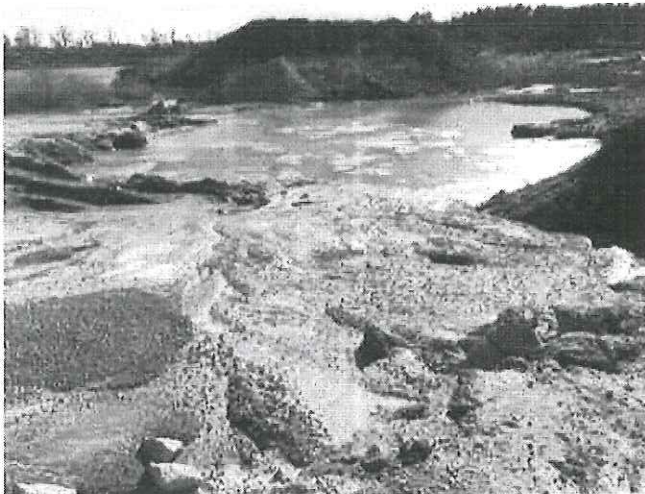
Photo 2: Please address the concrete washout area and implement a better management practice such as making sure the concrete is inert before it reaches the water or creating a forebay, etc. Please address within 30 days and submit photo documentation.
