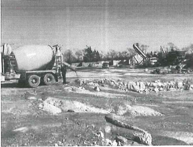
Photo 1: Please address the concrete washout area and implement a better management practice such as making sure the concrete is inert before it reaches the water or creating a forebay, etc. Please address within 30 days and submit photo documentation.
