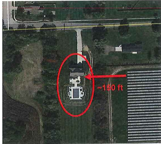
Dominion Indy III Solar Farm October 2016
