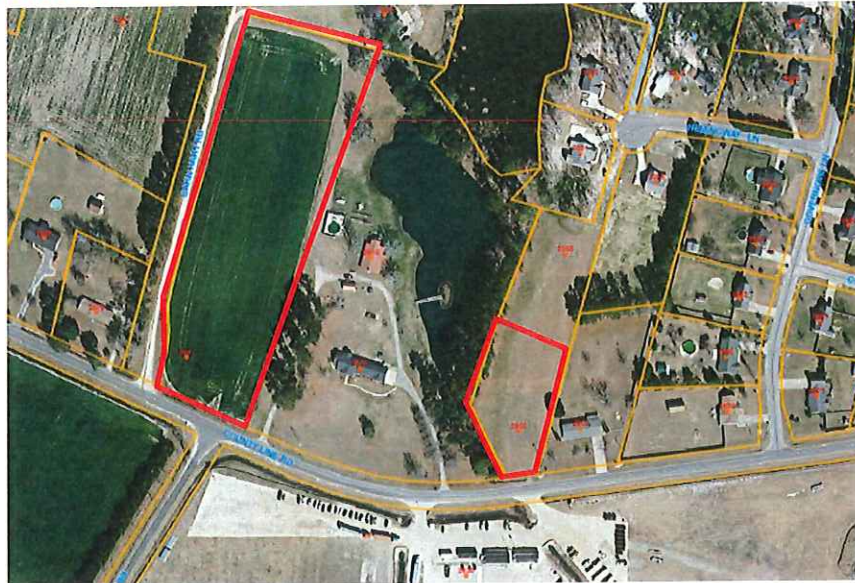
Innovative Solar 42 (2017) Cumberland County, NC
