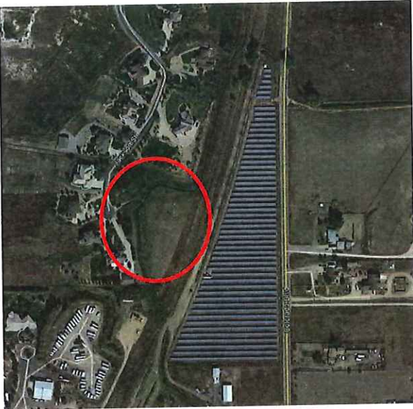
Brighton PV Solar, Adams County, CO June 2016
