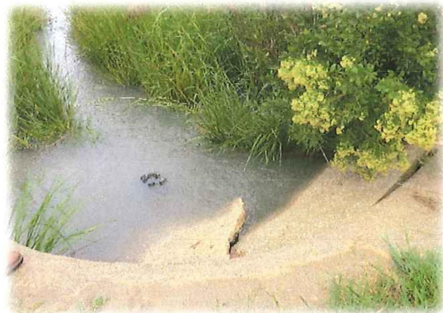
Collapsed headwall at River Road culvert during high tide, approximately 2,000 feet west of Chief Road (OO_04).
