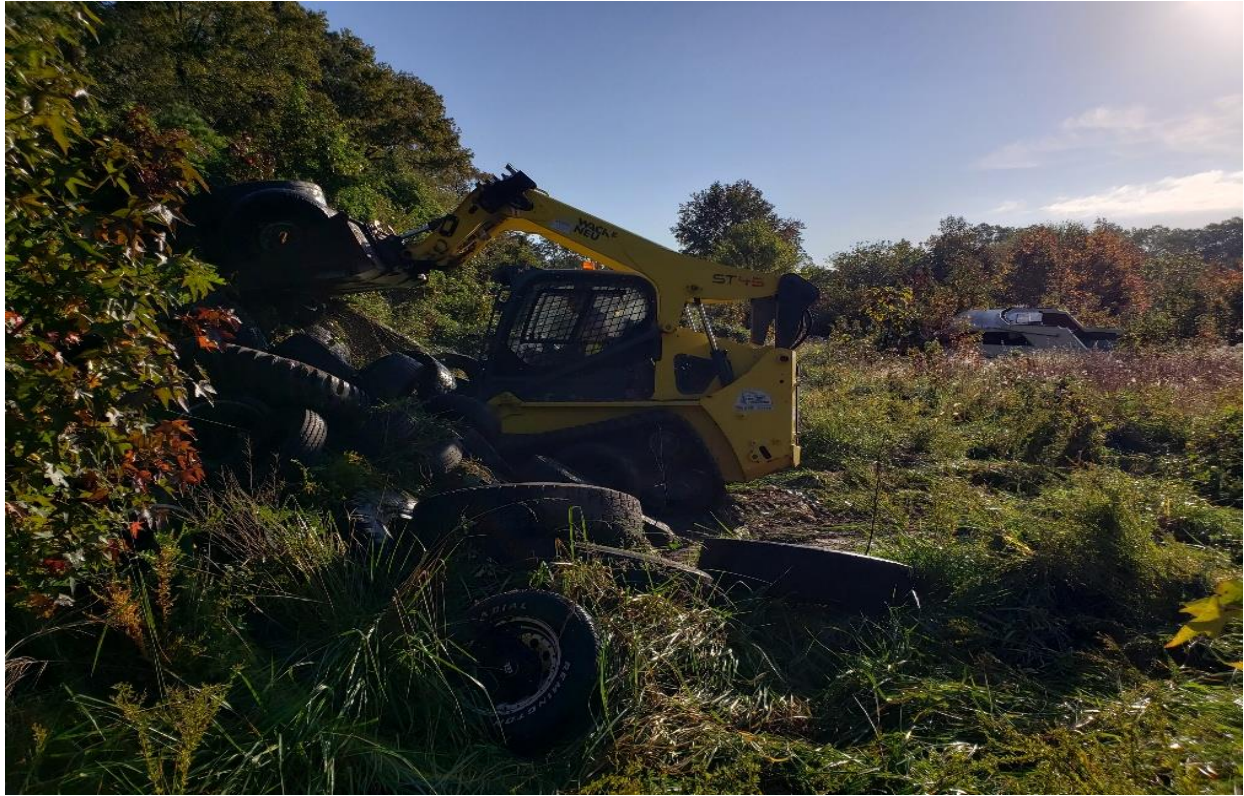
Excavation of tire pile in the east-central portion of the property.
