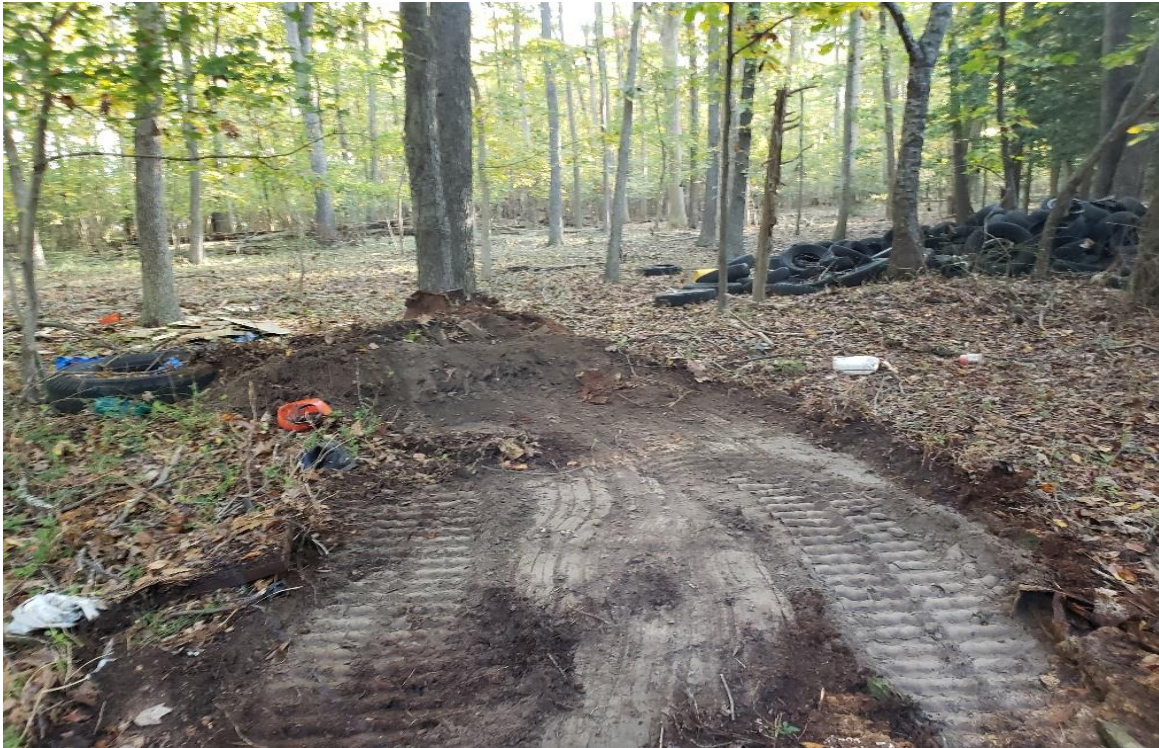
Excavation of small debris pile in the north-central portion of the property.
