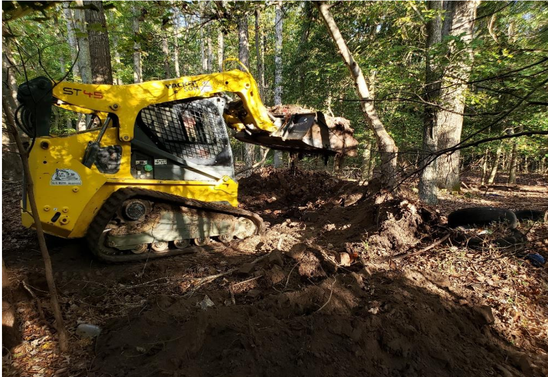
Excavation of debris pile in the northwestern portion of the property.
