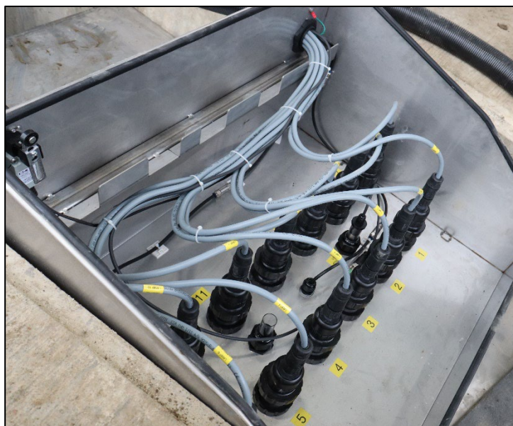
Figure 13: Enclosure Lamp Connections
