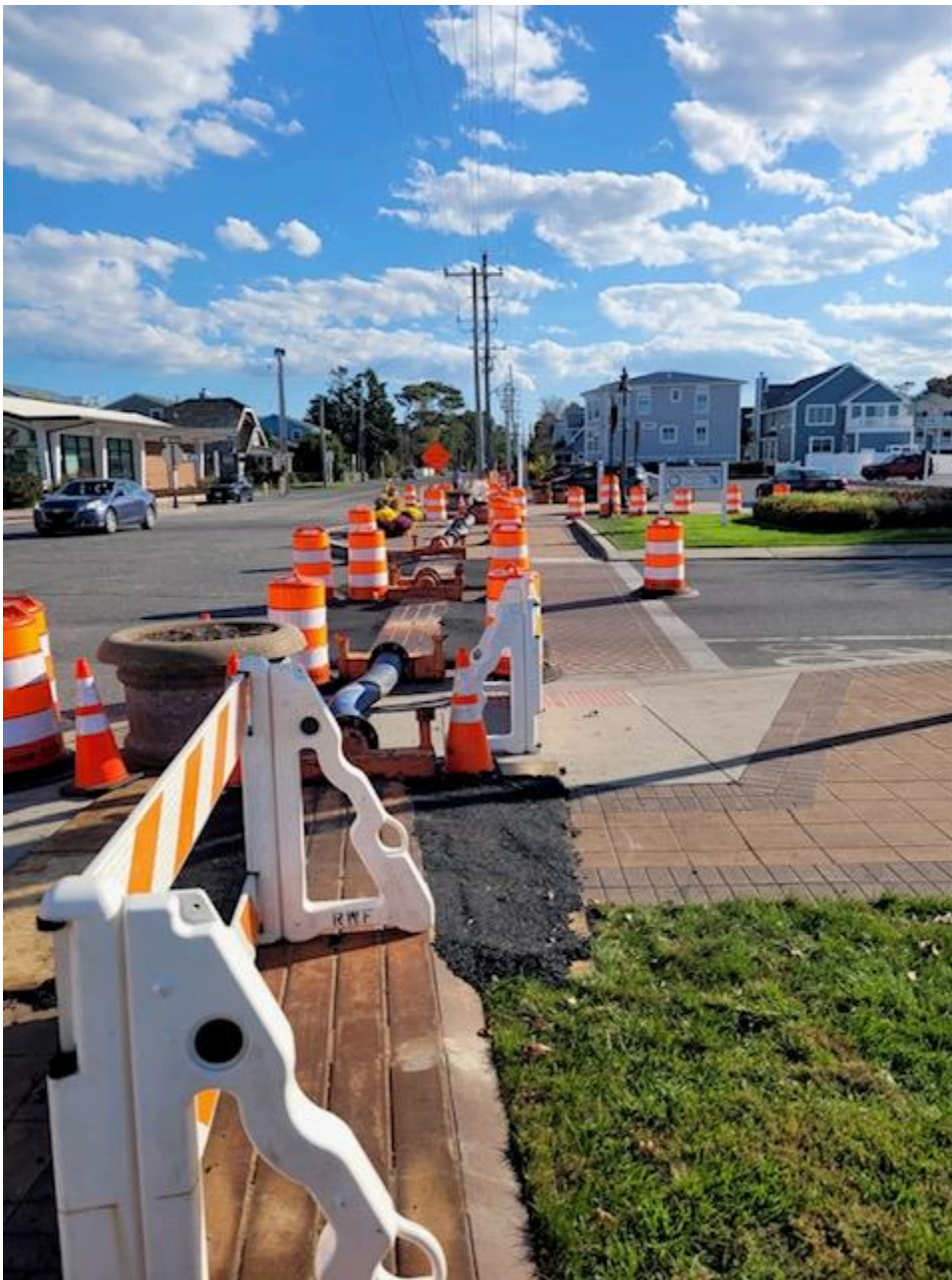
Garfield Parkway, Bethany Beach – Bypass Pumping Crossing
