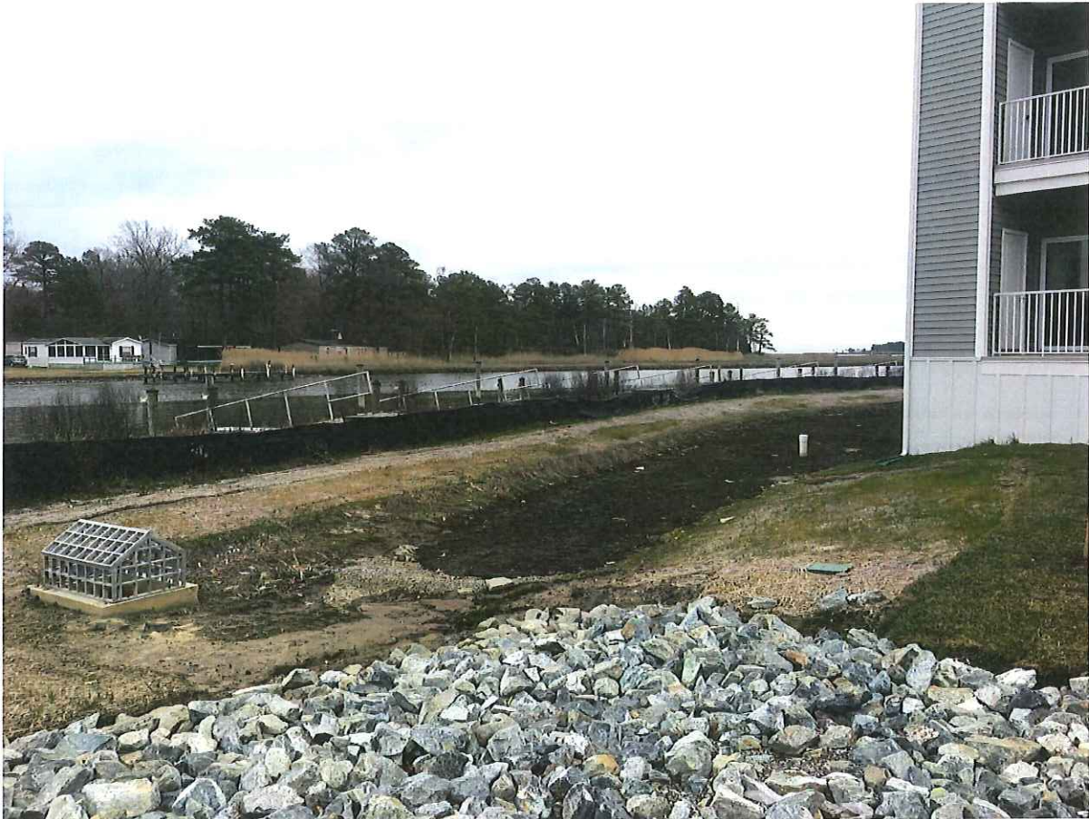
Dry stormwater detention feature in buffer on Love Creek.
