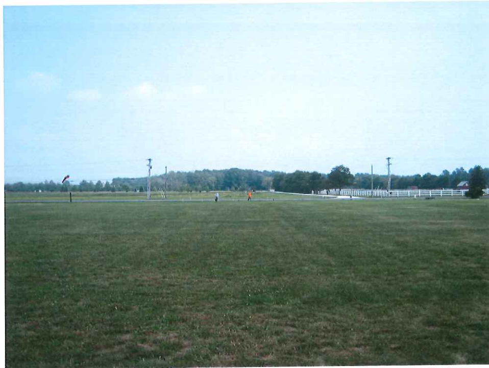
The power lines are buried at the end of the runway on Eagles Crest Road
