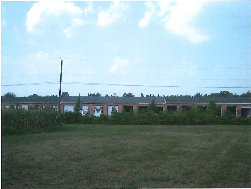
The runway end at Noxontown Road with the self storage buildings and unmarked power lines.
