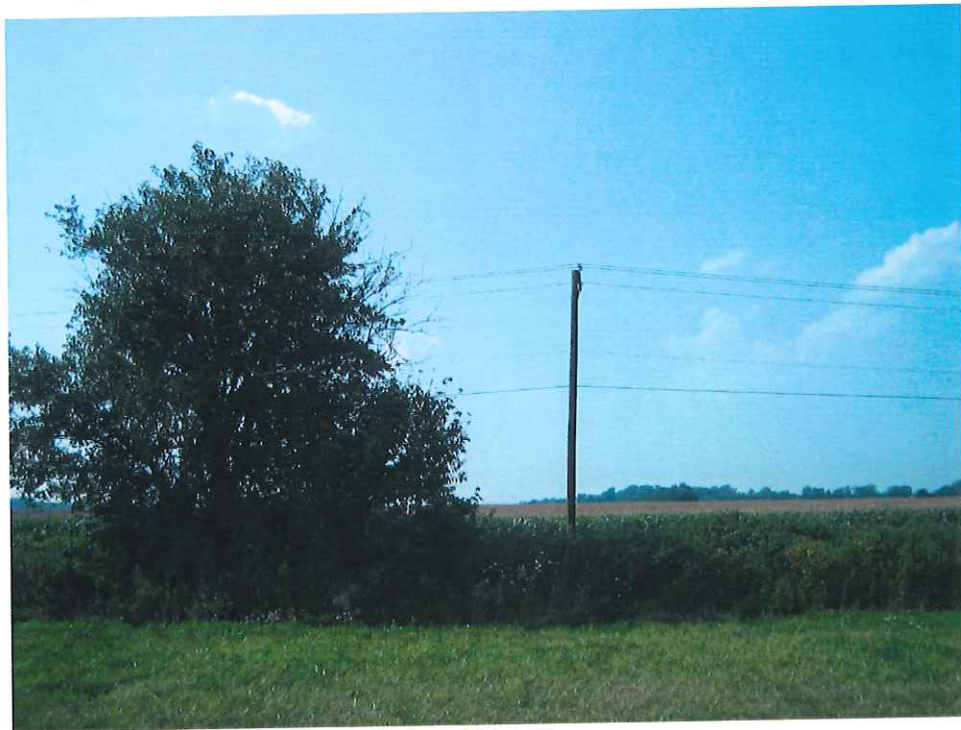
Closer look at the tree and power lines.
