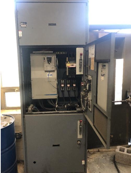
3. (3) RAS Pump VFD CPs located in Building PS-1
