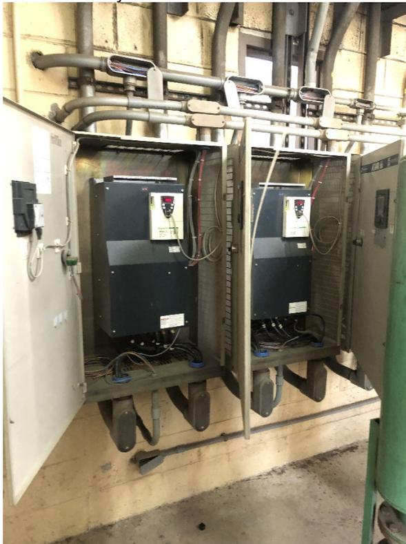
2. (3) Oxidation Ditch Blower VFD CPs located in Building B-3 Blower Room
