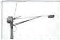
Cobra Head Light-Emitting-Diode (LED) Streetlight Style
