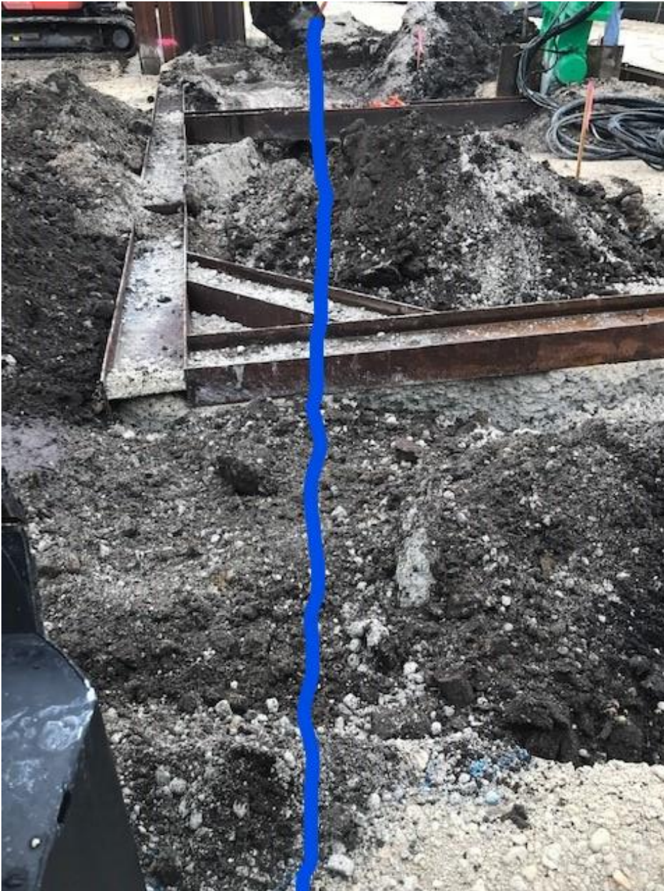
Approximate alignment of the municipal water main through the pump station excavation site
