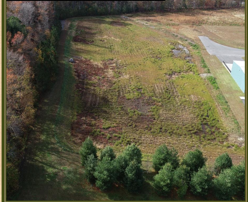
Delaware Coastal Business Park Ph 1 Dry Extended Detention Pond
