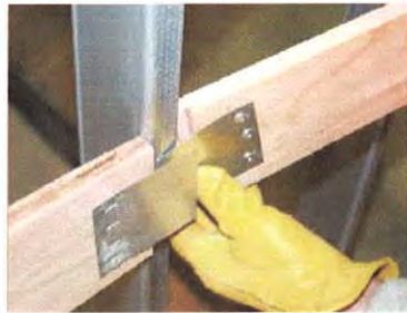
Overlap connector plates when using in long backing runs.
