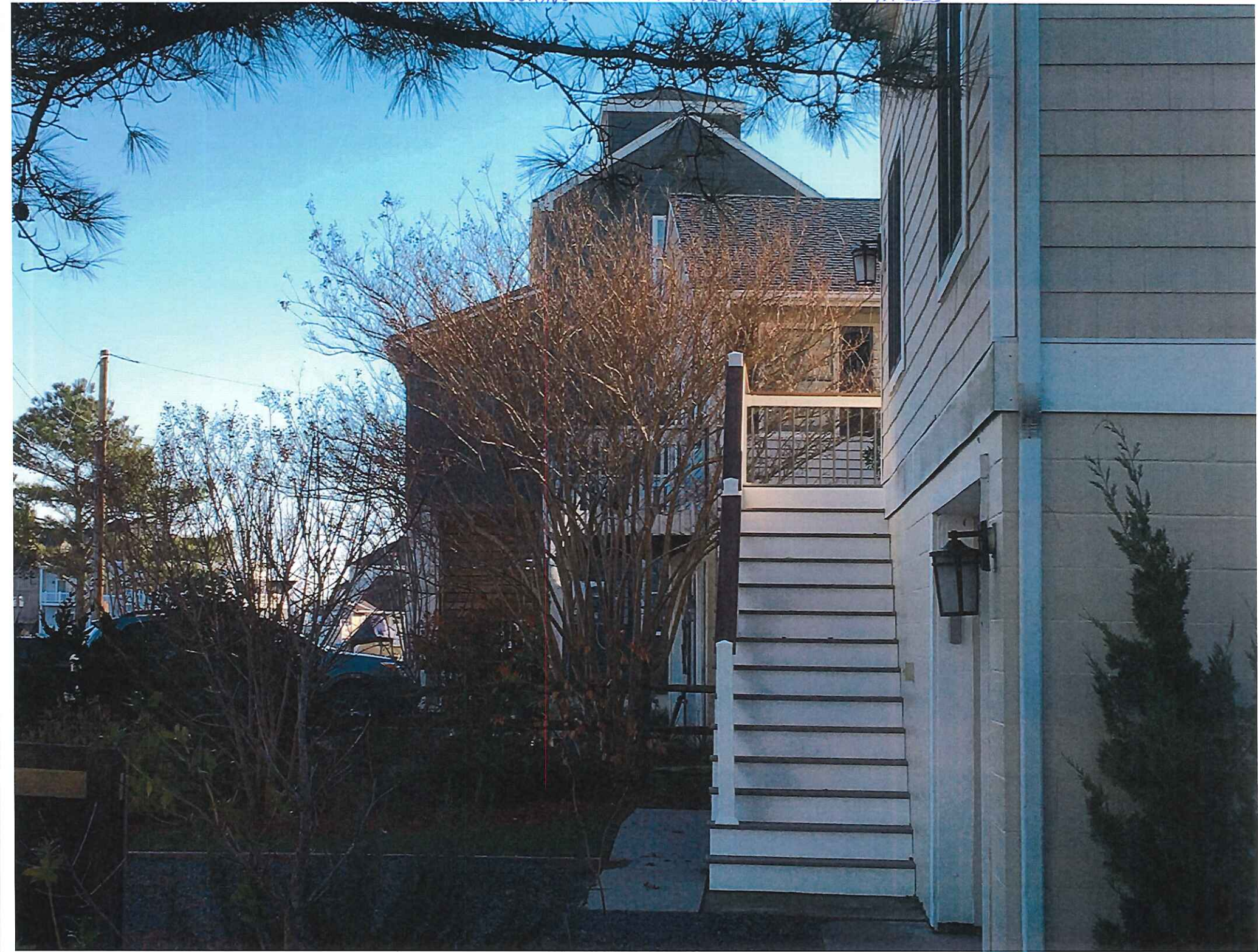
LOOKING SOUTH ALONG FRONT YARDS
