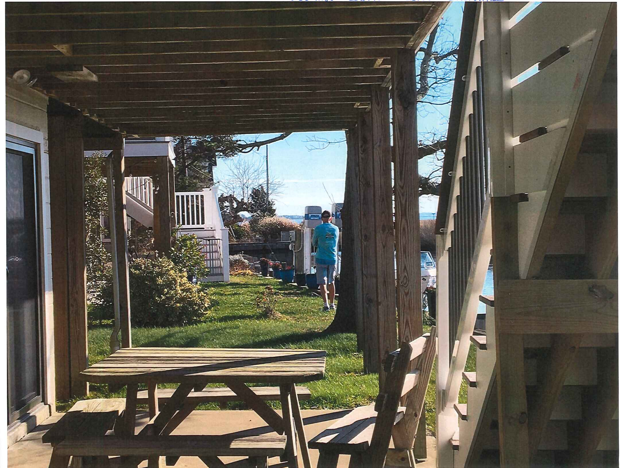
LOOKING SOUTH ALONG BACKYARD
